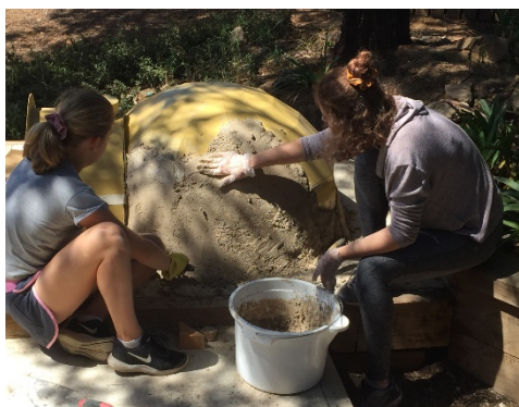
High School students hard at work building the new pizza oven near the Home Economics room
